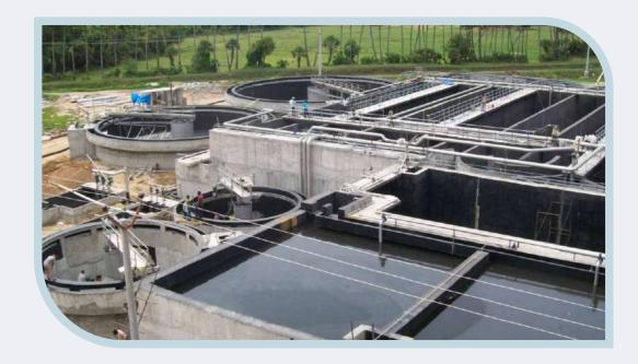
Onsite wastewater treatment, specifically the AG Series AWT plants, utilizes a concrete module with aeration, settling, and disinfection chambers in a closed pit. Ranging from 5 KL to 5 MLD capacity, these plants, housed in a separate room, minimize life cycle costs, accommodate varied tank shapes, and eliminate the need for long-distance wastewater transfer, efficiently returning purified water to its source.
